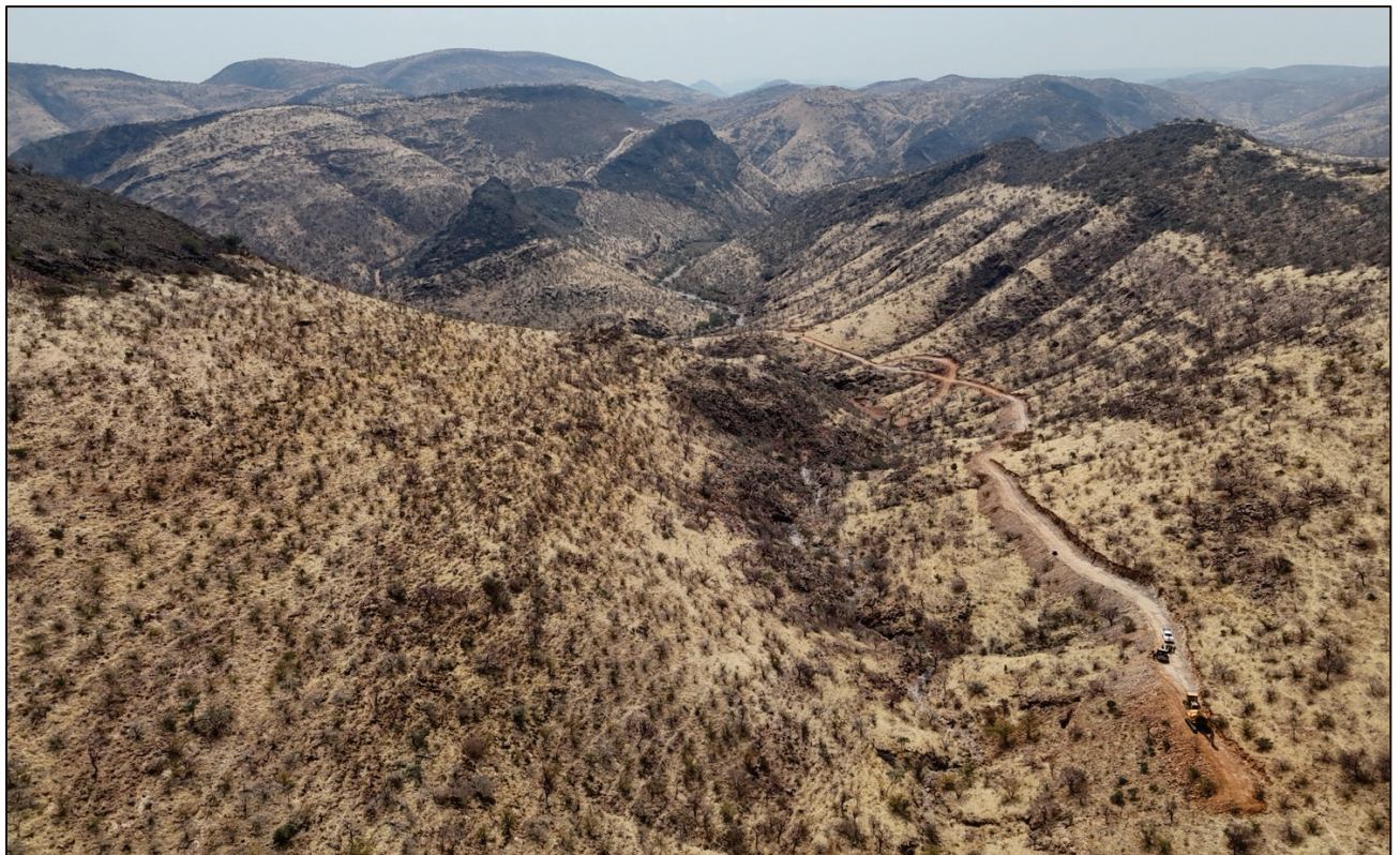
Figure 4 – KG Contractors building road to site DDOT007. Road to Donkey Hill in background.
