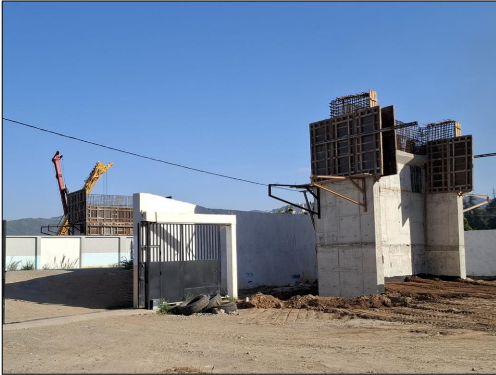
Figure 2: Construction of the access bridge over RN75
