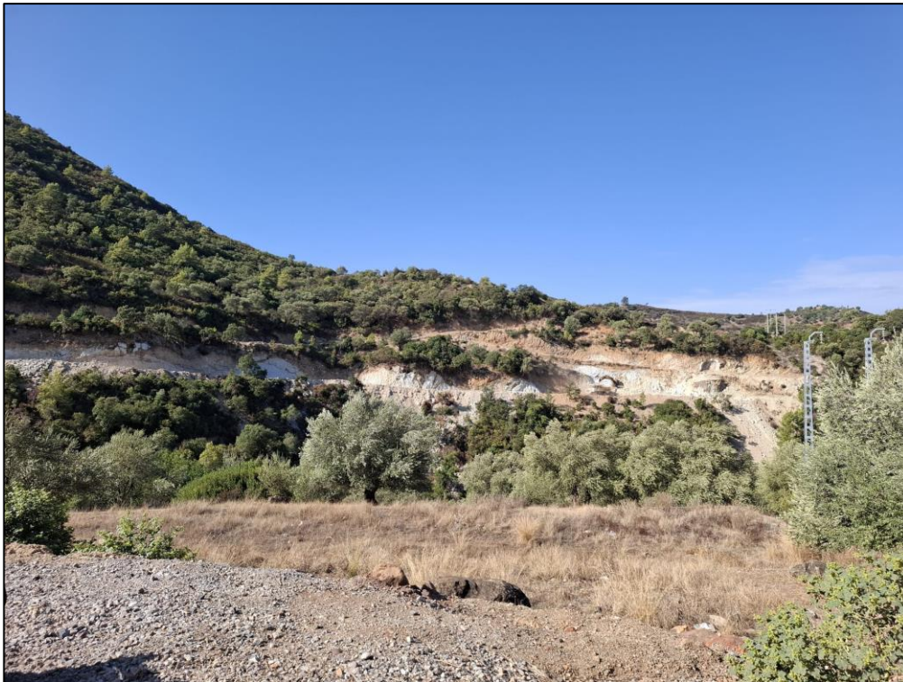
Figure 3: Site earthworks around the portal, with new electricity infrastructure in the left foreground
