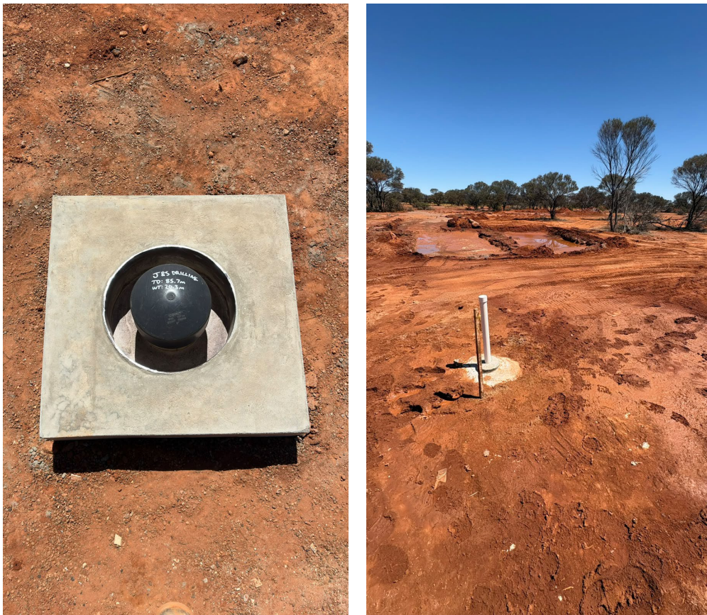
Figure 6. Water bore and monitoring bore at McNabs East completed in October. Testing has confirmed a suitable water source for mining requirements.
