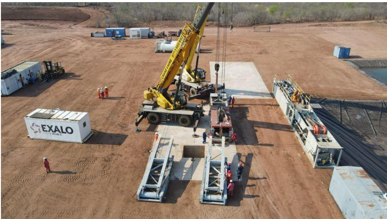
Figure 3 – Rig 202 substructure installation preparation
