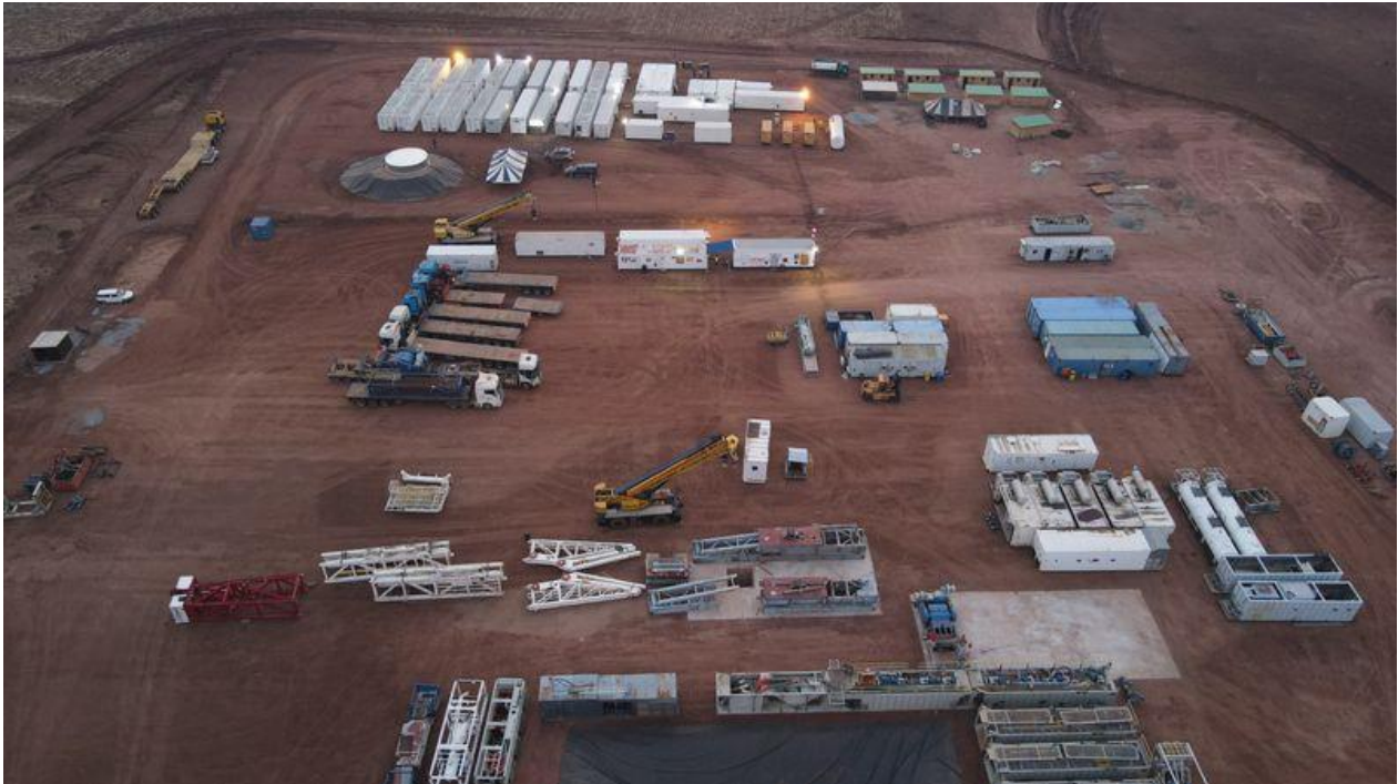
Figure 2 - Musuma-1 wellsite and rig camp aerial view
