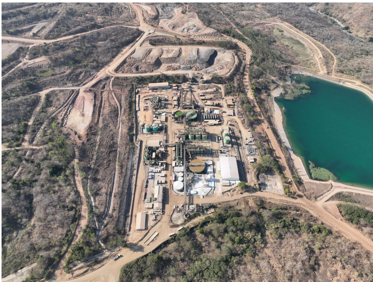
Figure 2: Kayelekera processing plant and ROM stockpile area, September 2026.
