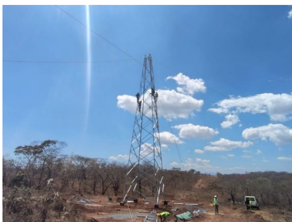
Figure 6 and Figure 7: Tower erection and installed transformer at Kayelekera
