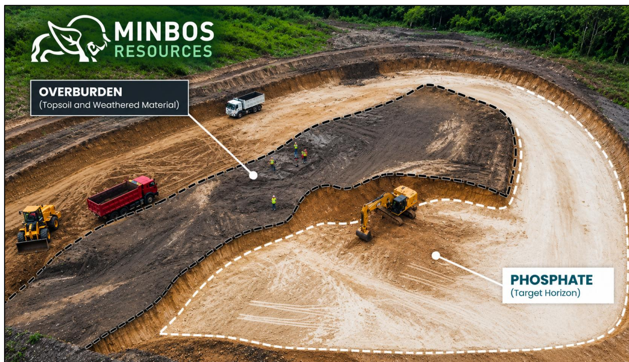
Figure 3: Technical and operational supervision teams overseeing pit benching, material handling, and truck loading operations.
