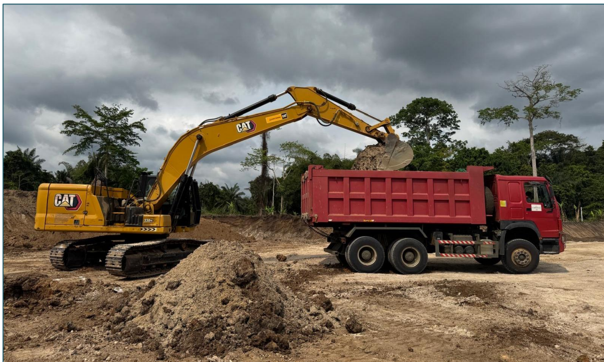
Figure 4: Active excavation and direct truck loading of first mined phosphate ore at the Cacata pit face.
