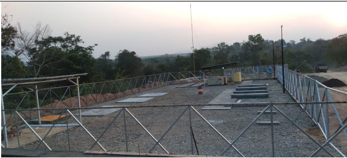
EPF Civil Work
