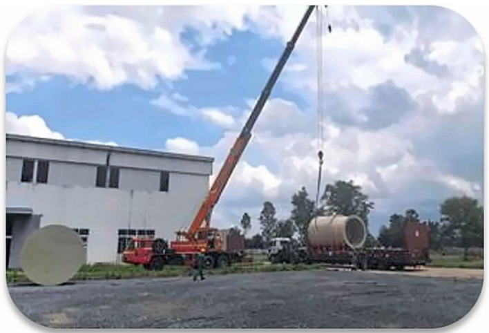
Figure 2 Unloading and handling of process vessel
