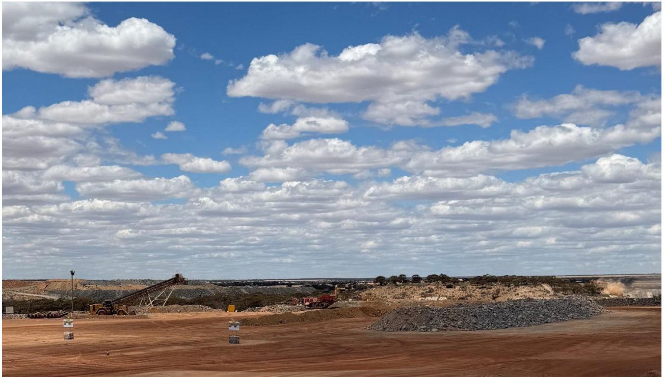
Figure 6: Edna May ROM Stockpile (October 2026)
