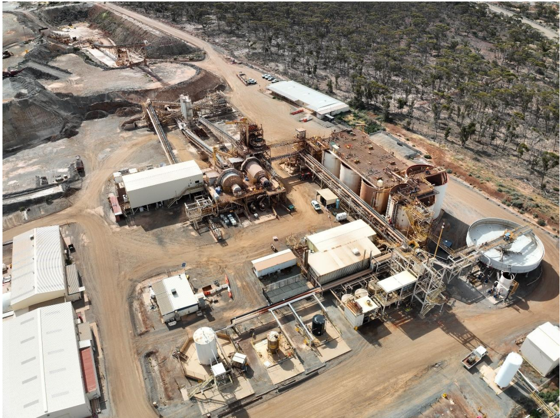
Figure 2: Edna May Processing Facility
