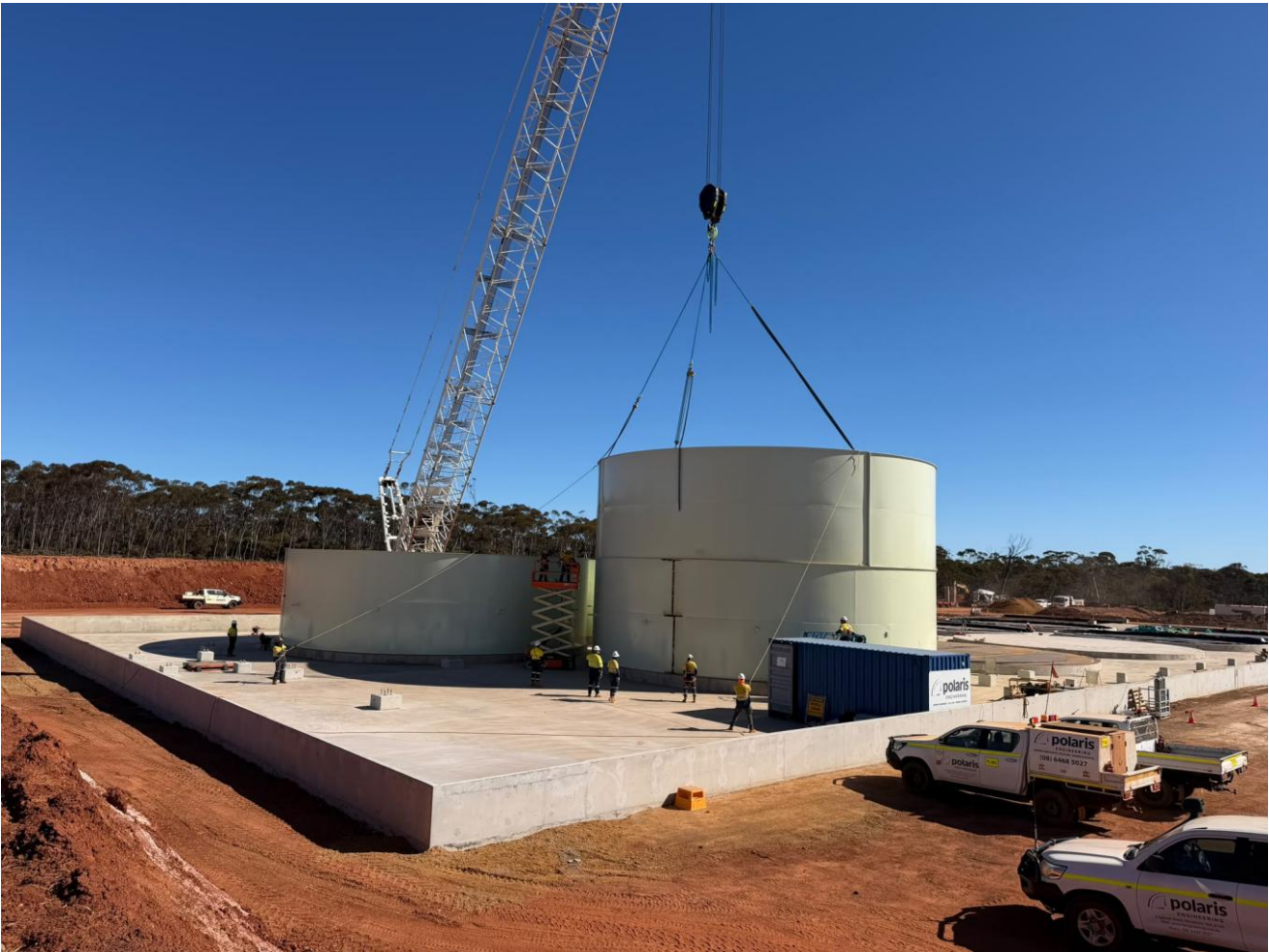
Figure 8: CIL Tank Installation – Lake Johnston
