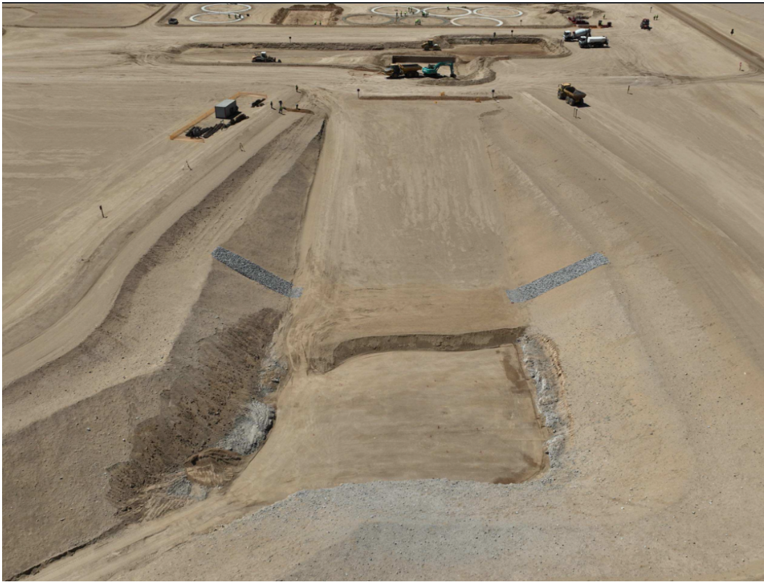
Figure 4: Run-of-Mine bin excavation and retaining wall preparations (October 2026).
