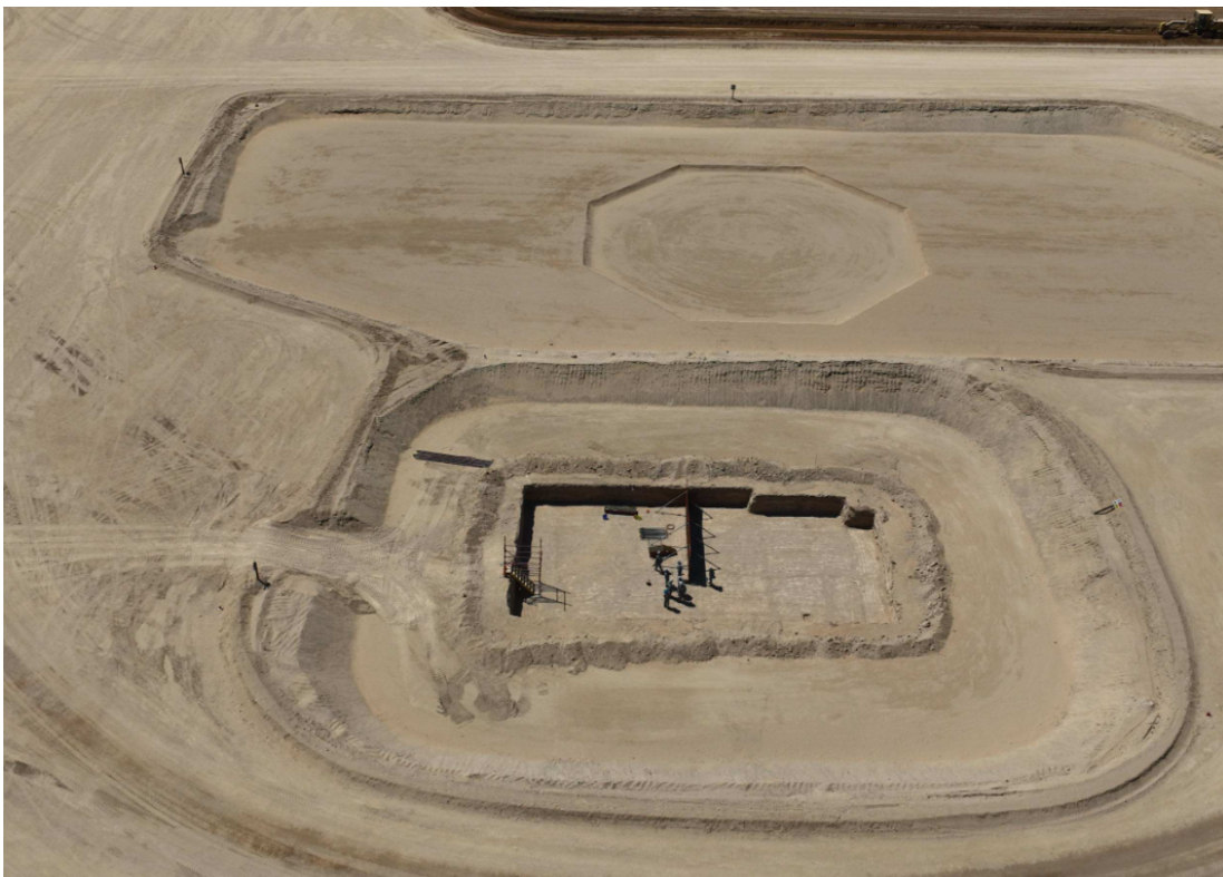
Figure 5: Fine and coarse mill foundation preparations (October 2026).
