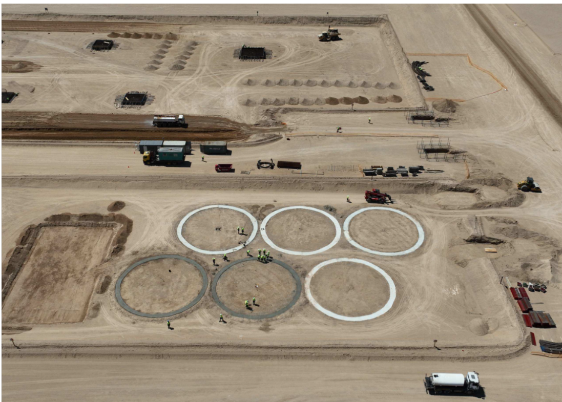
Figure 3: Leach tank ring beam preparations (October 2026).
