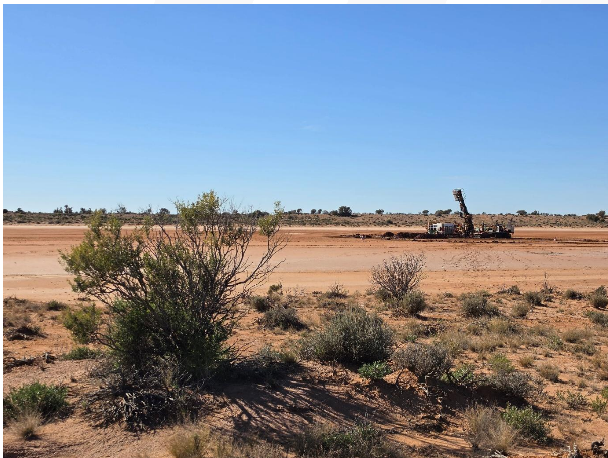
Plate 3: Drilling rig on the lake
