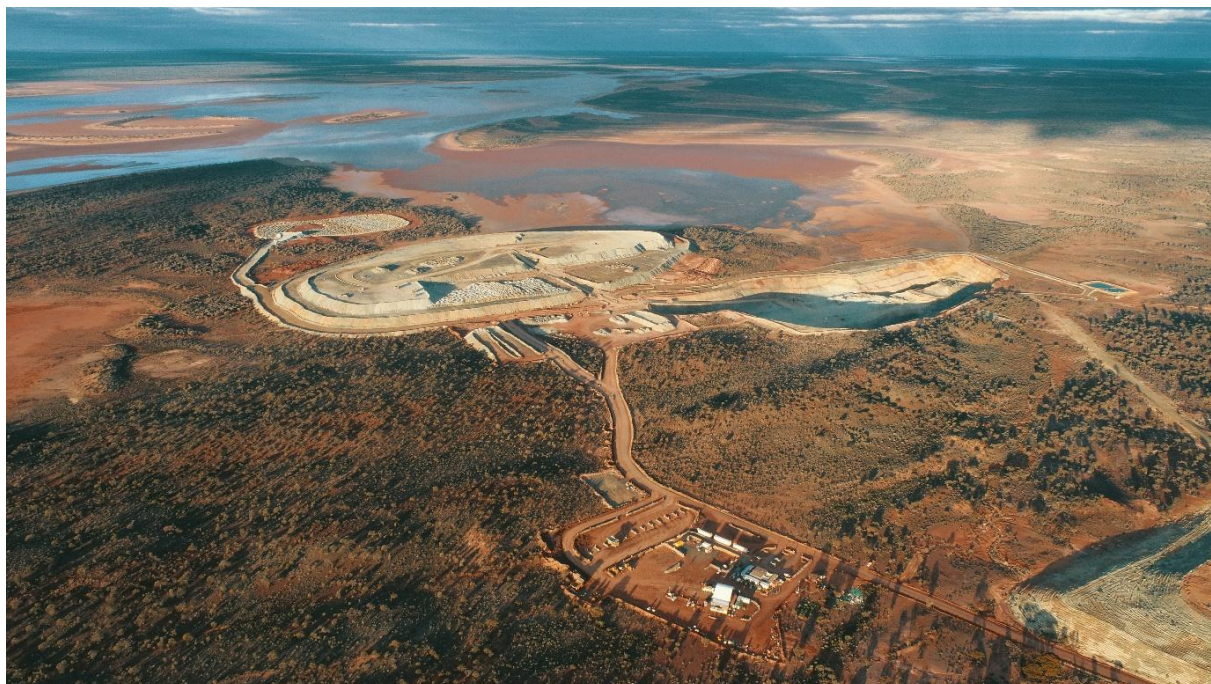
Plate 1 - Devon Pit Gold Mine – Photo taken 4 July 2026
