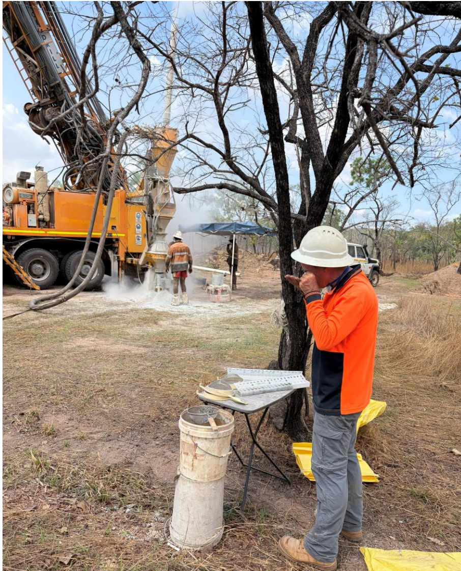
Figure 3: RC Drilling currently underway at the Berinka Pine Creek Gold-Copper Project
