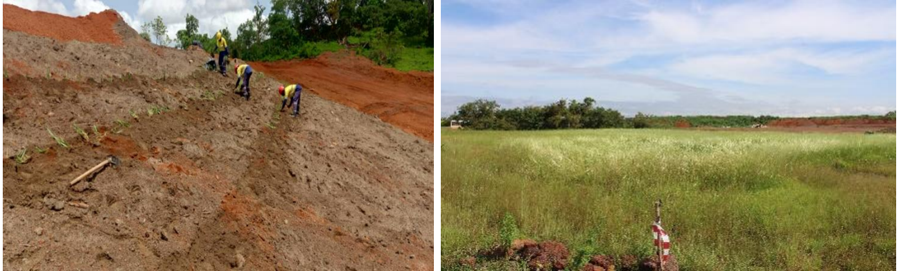
Figure 16: Stabilisation and Erosion-Control Works at Water Storage Dam and Figure 17: Environmental Monitoring
