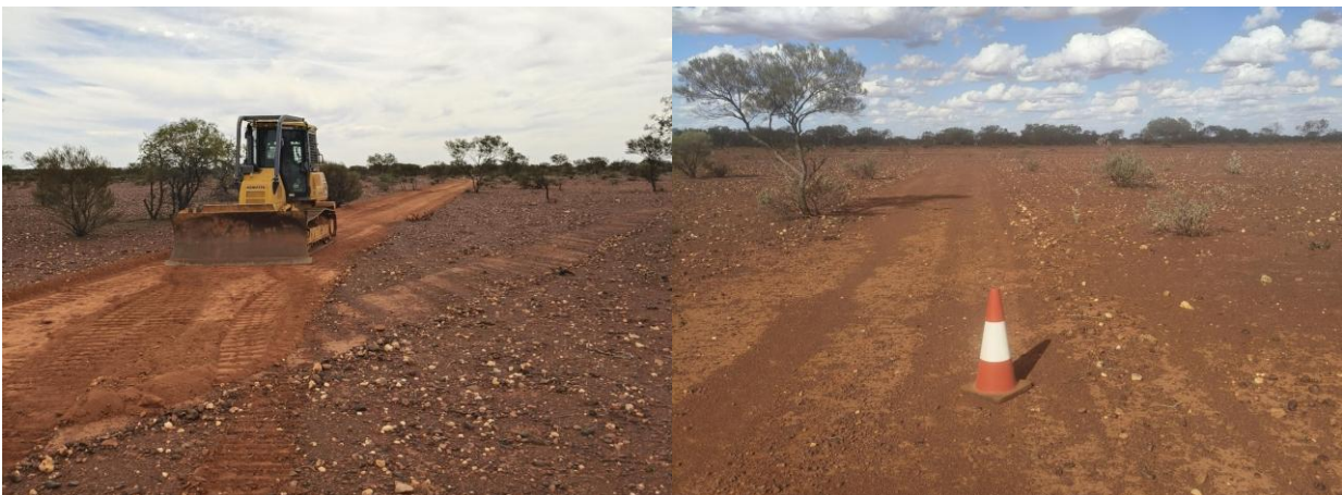
Figure 2 and 3: Access track clearing along a drill fence line and Cleared fence line with collar marker, Lady Alma
