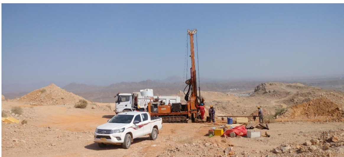
Figure 36 – Drill site set in progress at MDO site
