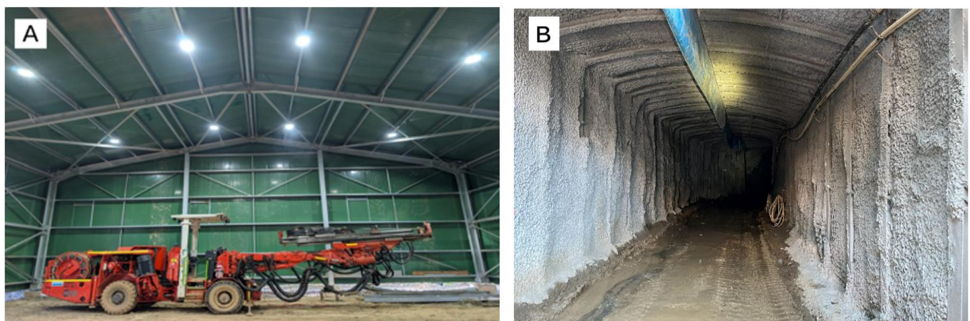
Figure 1 - Photos of the Dittmer mine development. (A) Completed acoustic shed; (B) Upgraded level 4 underground access development to provide access for underground extension drilling and trial mining.
