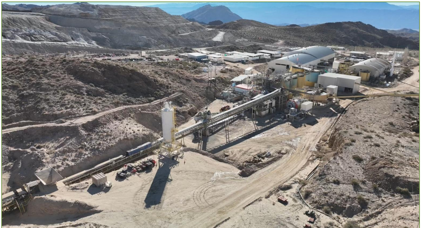
Casposo Processing Plant
