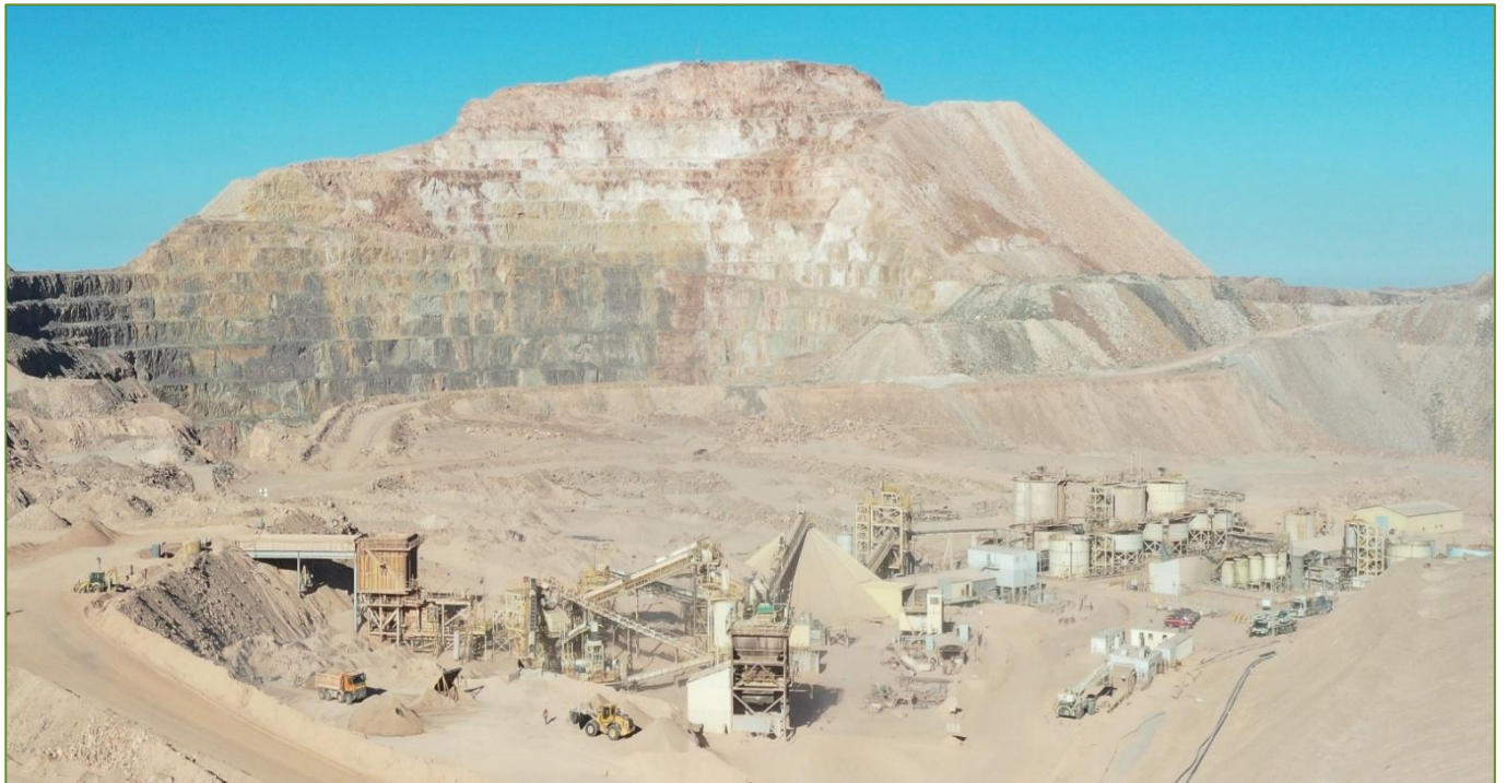
Guanaco Processing Plant
