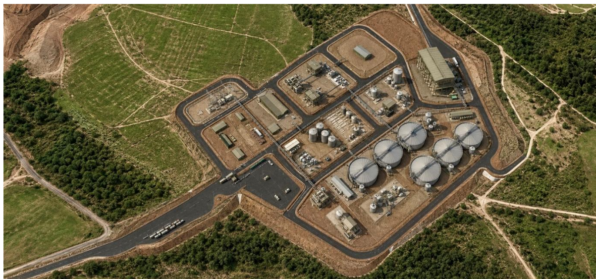
Figure 1: Overall Process Plant Layout – Looking North.
