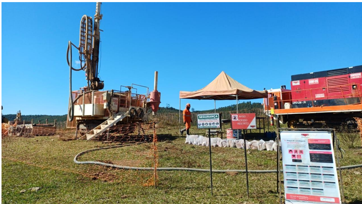
Figure 10: Drilling activities during the September 2026 quarter.
