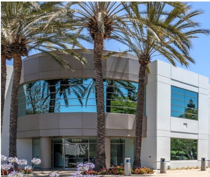
NEW LUMOS FACILITY · CARLSBAD, CALIFORNIA
