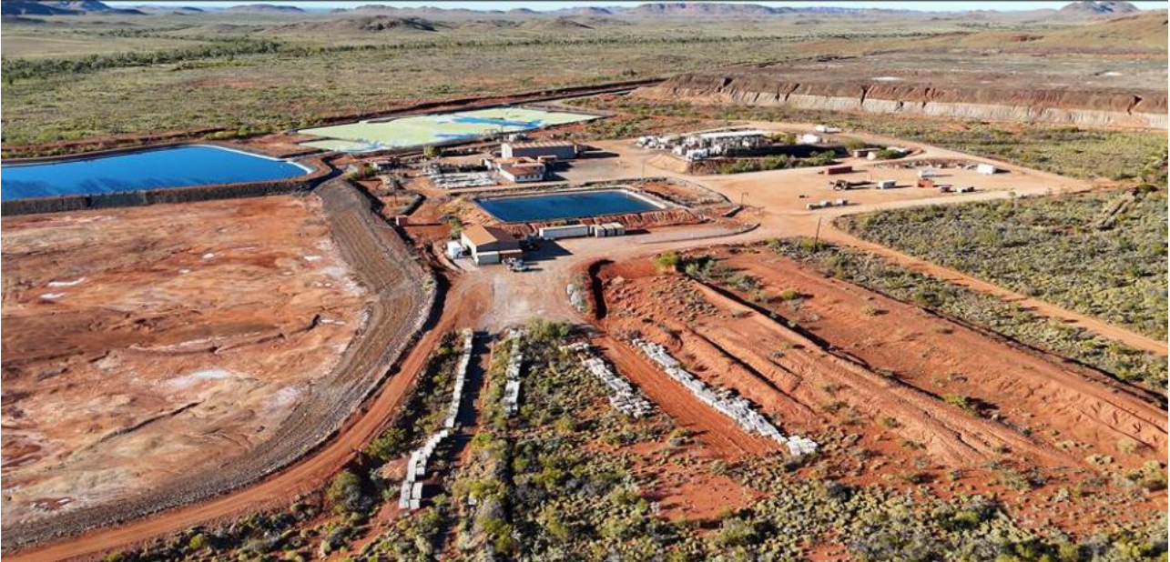
Figure 2: Whim Creek site including permitted heap leach infrastructure. Source: ASX announcement, 3 September 2026.
