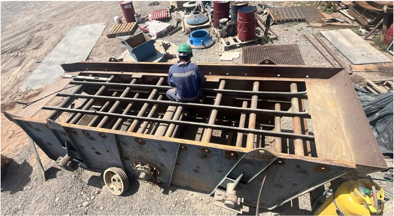
Image 4: Three-deck screen refurbishment works underway.
