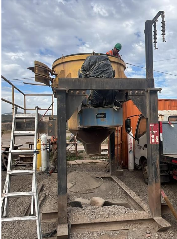
Image 2: refurbishment works underway on second vertical shaft impact crusher (VSI)
