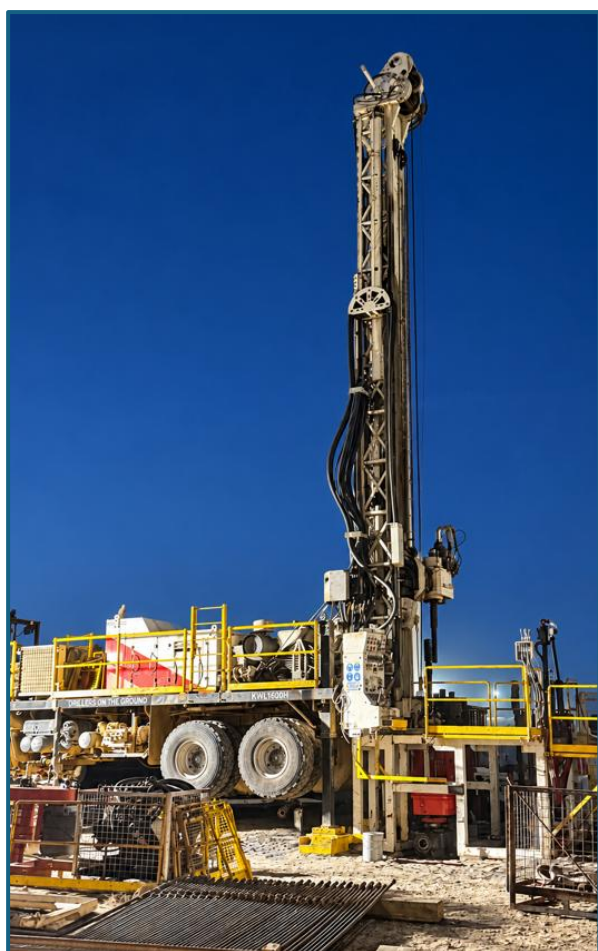
Figure 1: Workover rig on location at LF-03
