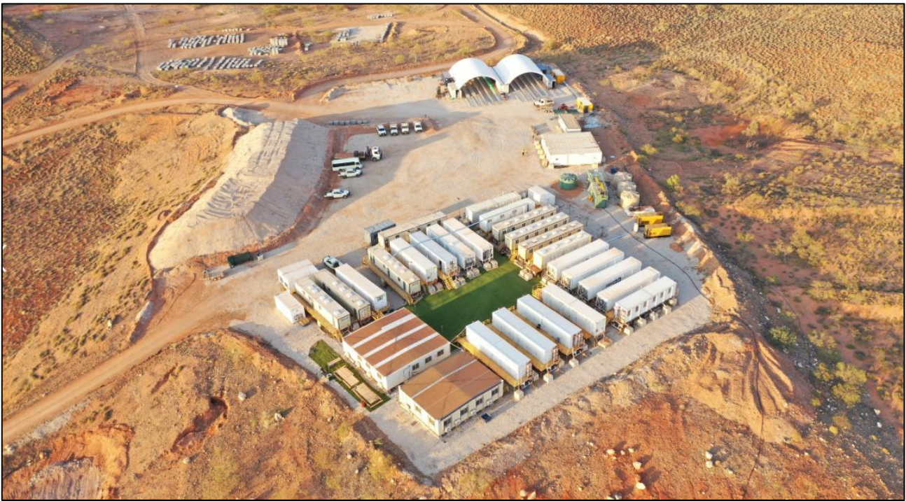
Plate E.1 Early works camp
