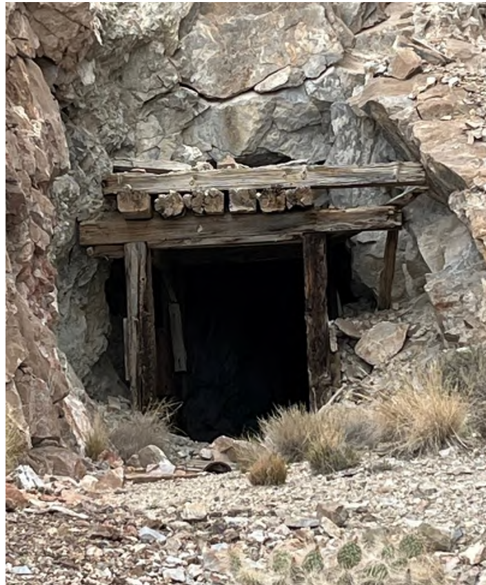
Figure 1- Bureau of Mines Adit- Cupric Prospect
