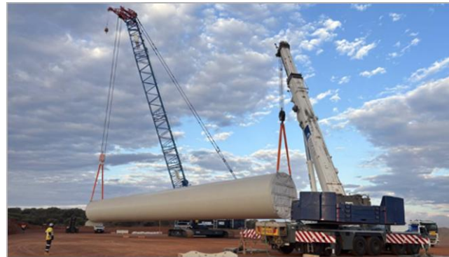
Wind turbine tower section lift
