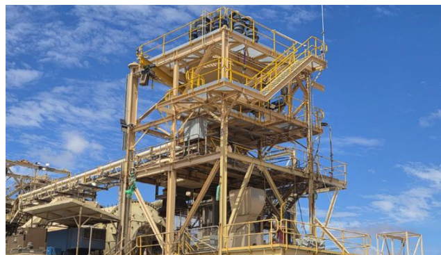
New cyclone tower structure in place
