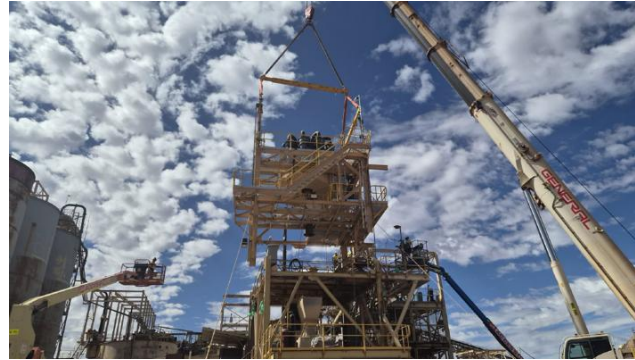
Lifting new cyclone tower
