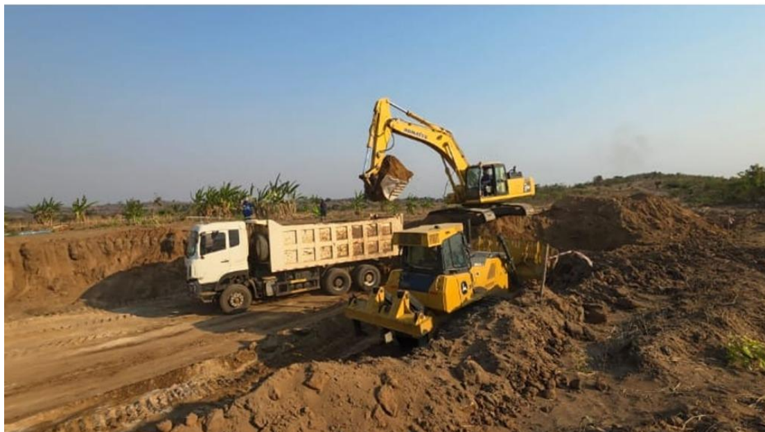
Image 2: Hydraulic excavator, vibratory roller and dump truck working in tandem to excavate and develop the mining pit at Kanyika.
