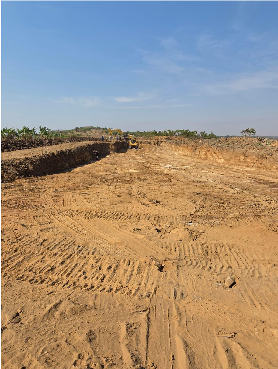
Image 1: The completed pit number 1
