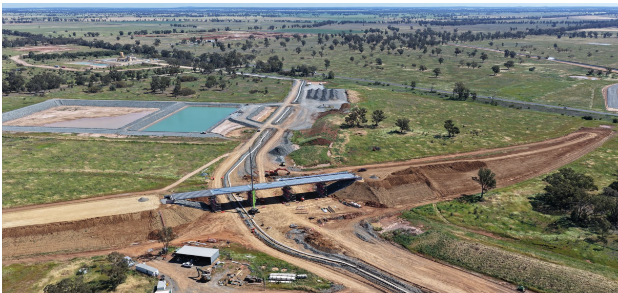
Kyalite Bridge Works Overview (29/09/26) – looking south
