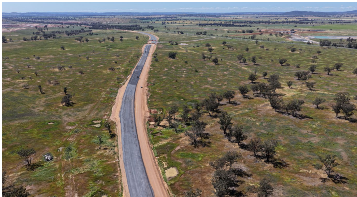
Roadworks (looking North)
