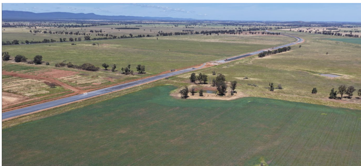
Roadworks (looking South)
