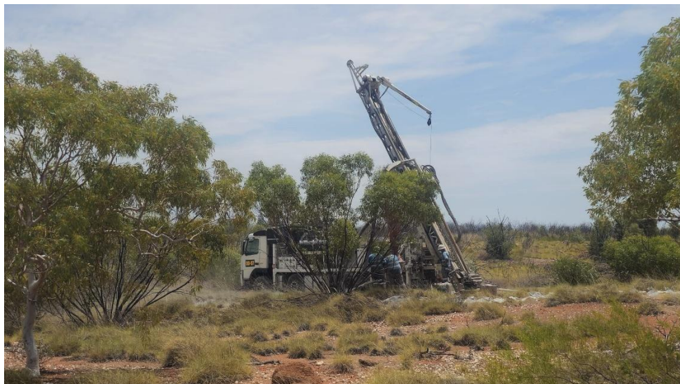
Figure 1 Sybella drilling in progress
