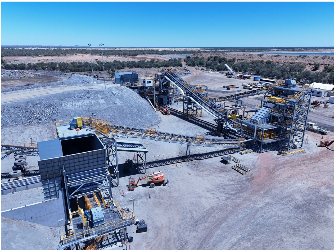
Photo 2. Construction progress – ROM bin, crusher and screening areas. Operational post Quarter end.
