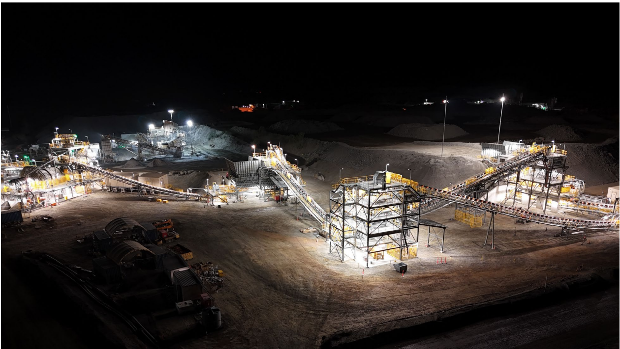
Photo 4. Construction progress – the new processing facility at night.
