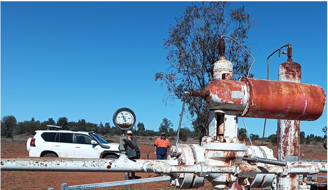
Figure 2 Managing Director Kane Marshall with operations personnel inspecting the Major-4 wellhead facilities as part of discussing operating protocols for bringing the Major Gas Field onstream.
