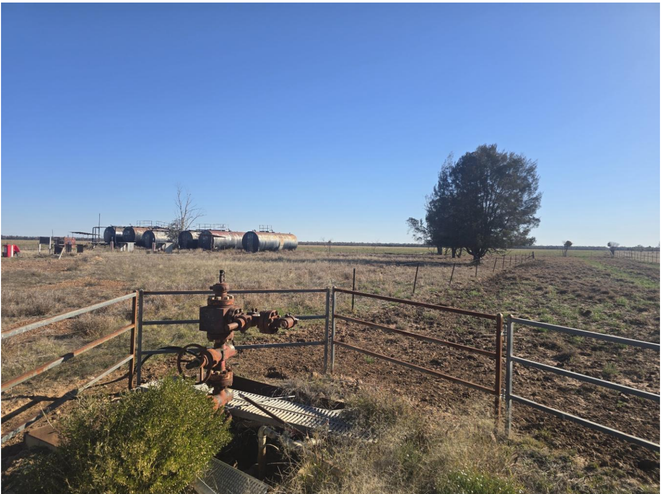
Figure 3 Looking east the Riverslea tank farm where installation of new load out pump and skimmer tank is planned for next quarter.
