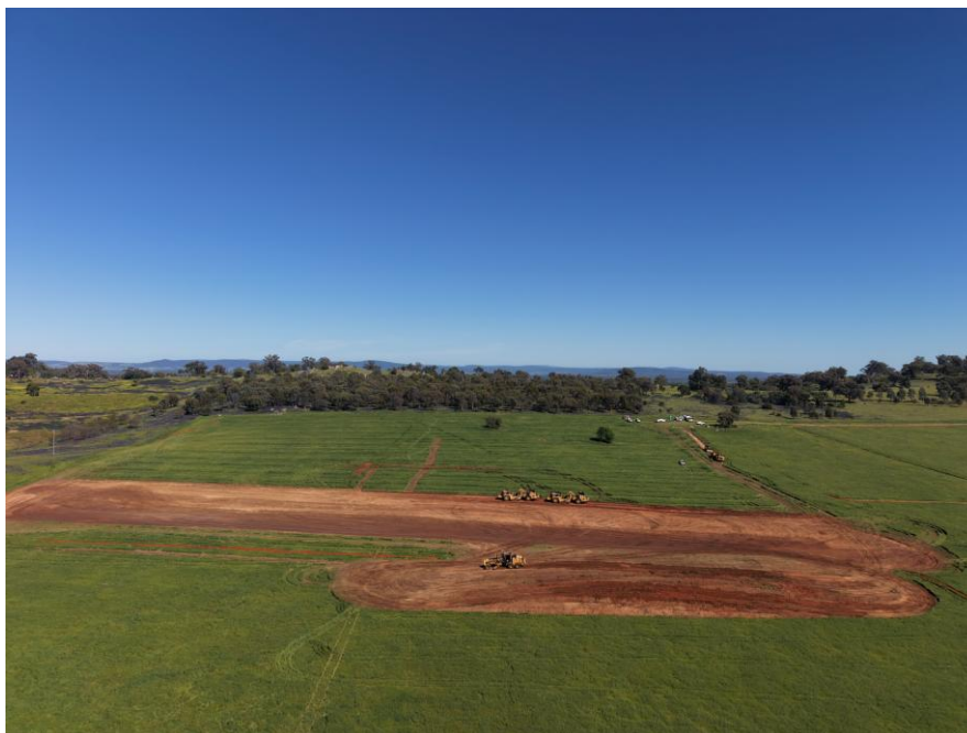
Civil earthworks underway at Villa Estate-Cowra.
