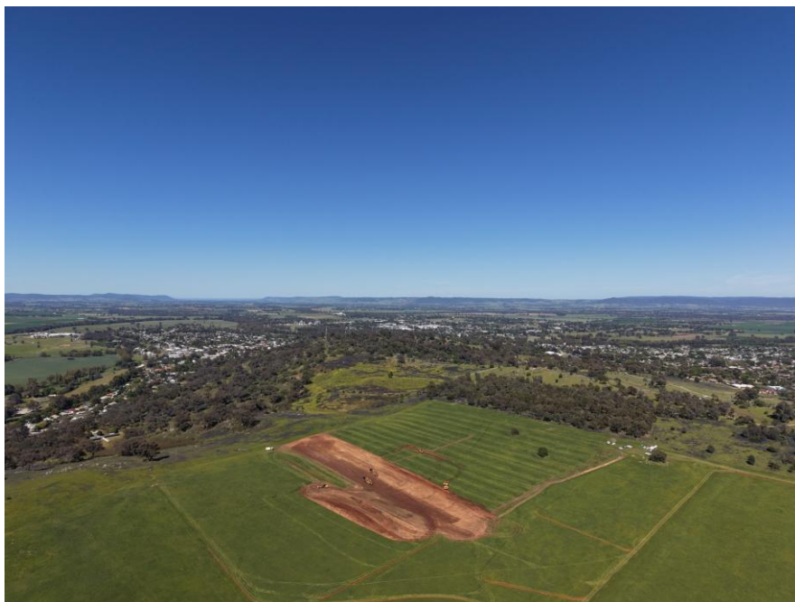
Aerial view of the Villa Estate site and Cowra township.
