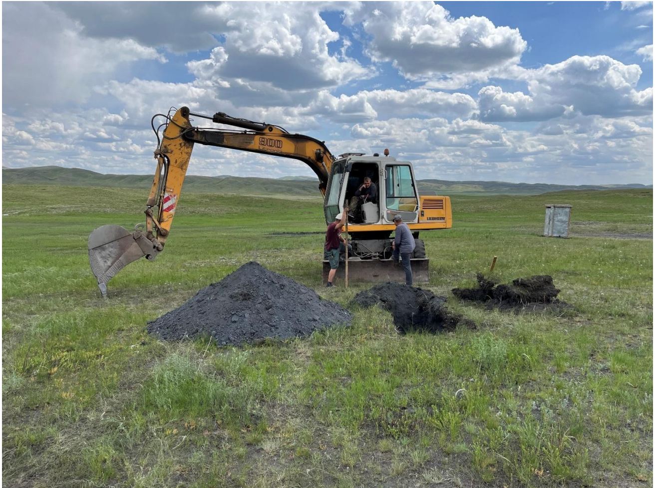
Figure 9 - Exploration test pit illustrating soft friable nature of the graphite mineralisation
