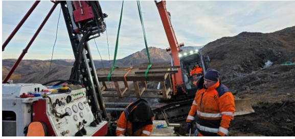
Rig operations at Grønnedal
