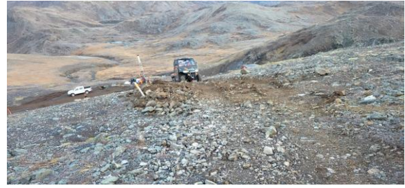
Site access and preparation supporting the campaign
