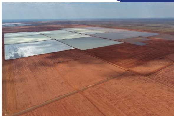
Figure 4: Crystalliser pond lining and filling
