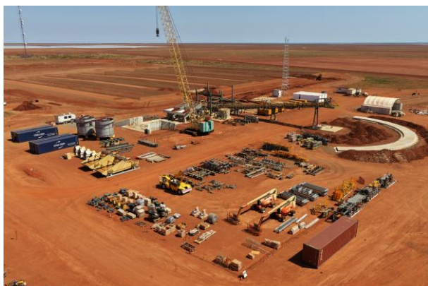
Figure 3: Salt wash plant construction
