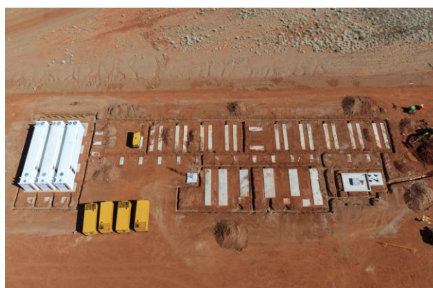
Figure 6: Stockyard conduit installation
