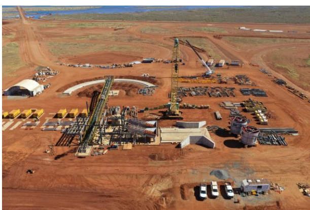
Figure 5: Salt wash plant installation
