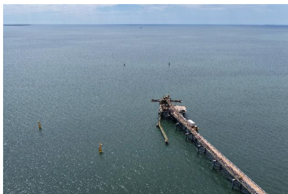
Figure 7: Navigation aids installed at the Port of Mardie
