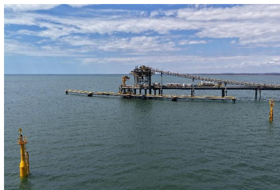
Figure 8: Jetty Head including catwalks, berth and mooring piles
