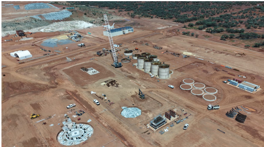
Figure 5 – Youanmi Processing Plant construction
