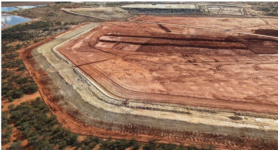
Figure 6 – Youanmi Tailings Storage Facility earth works
