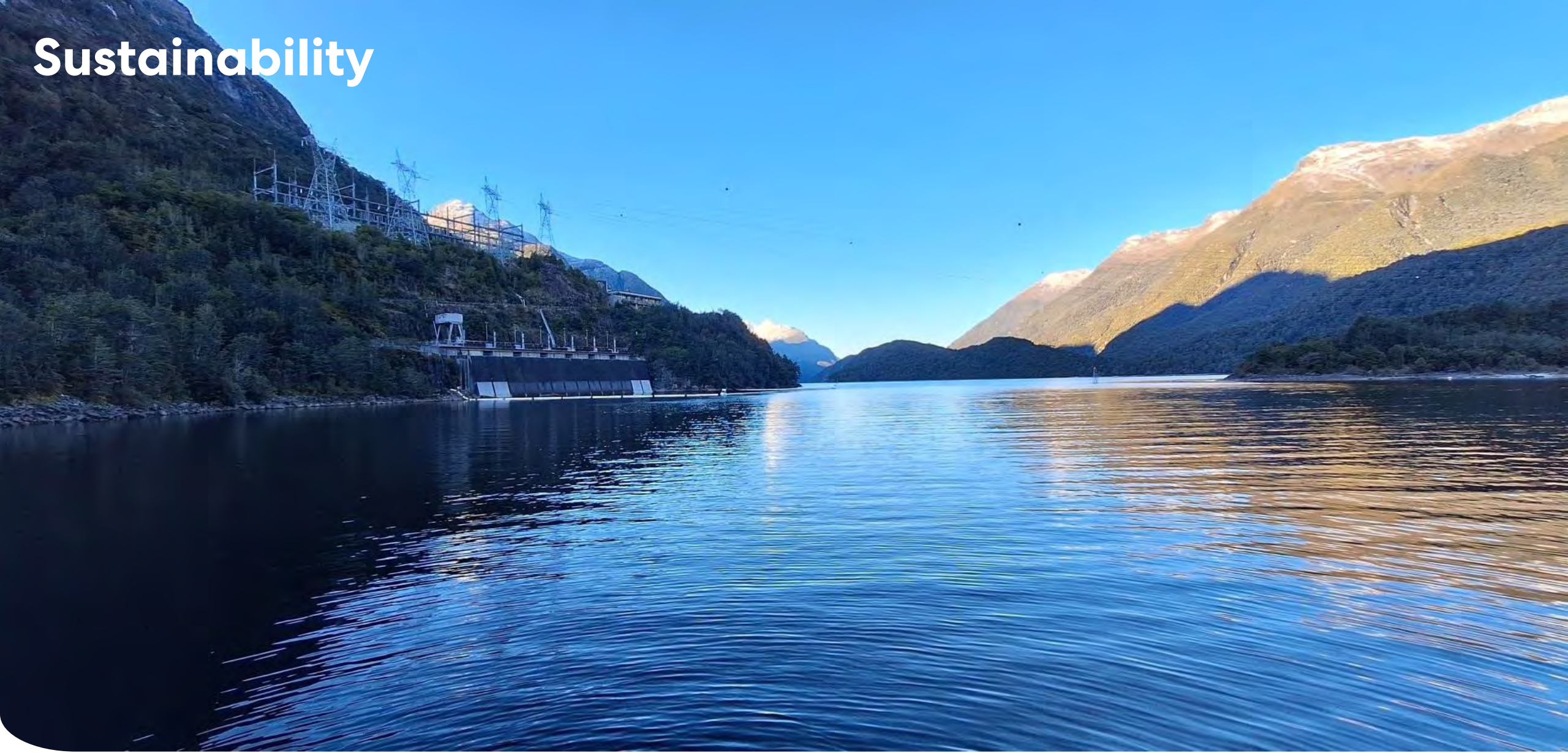
Manapōuri Power Station in Fiordland National Park.
