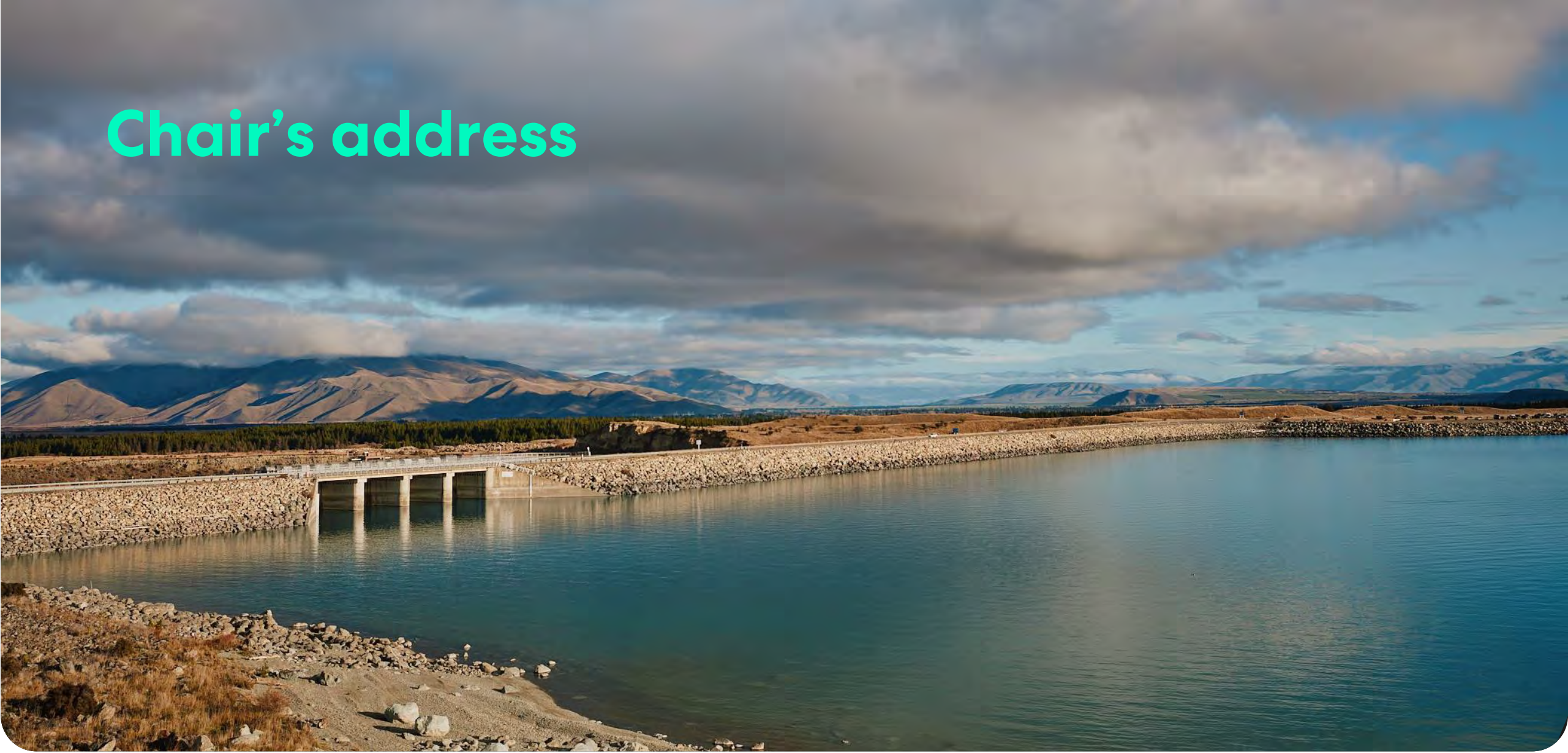
Control structure and spillway, Lake Pūkaki, South Canterbury.
