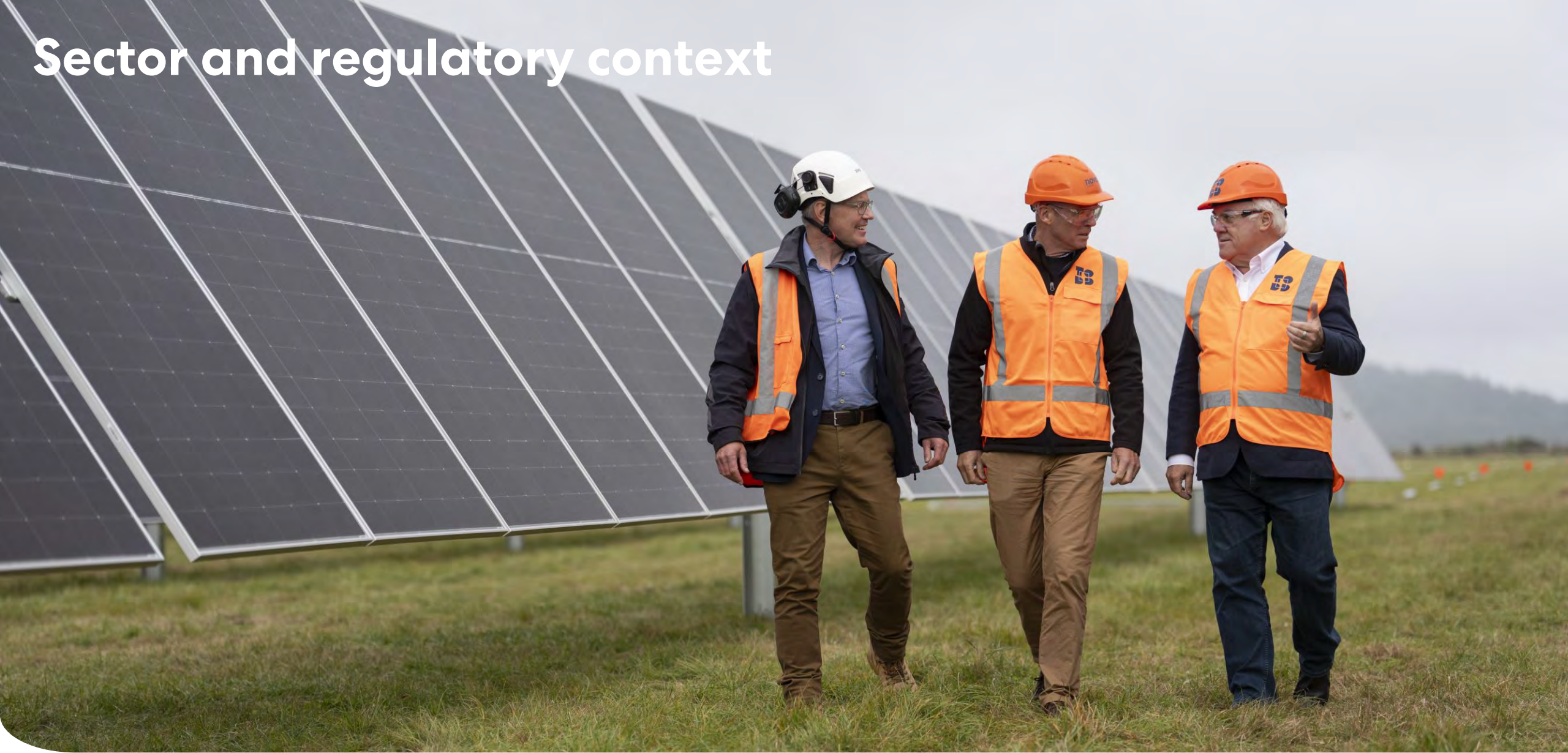
First row of panels at the Meridian and Nova Energy joint venture Te Rahui Solar Farm near Taupō.
