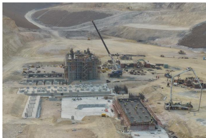
Photo: Broader civil works footprint nearing completion for first kiln installation and associated infrastructure.
