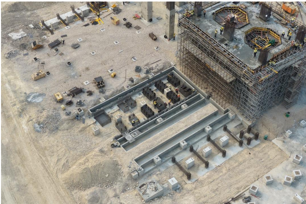
Photo: Kiln foundations and table-top deck to support large-scale mechanical combustion kilns ahead of erection.
