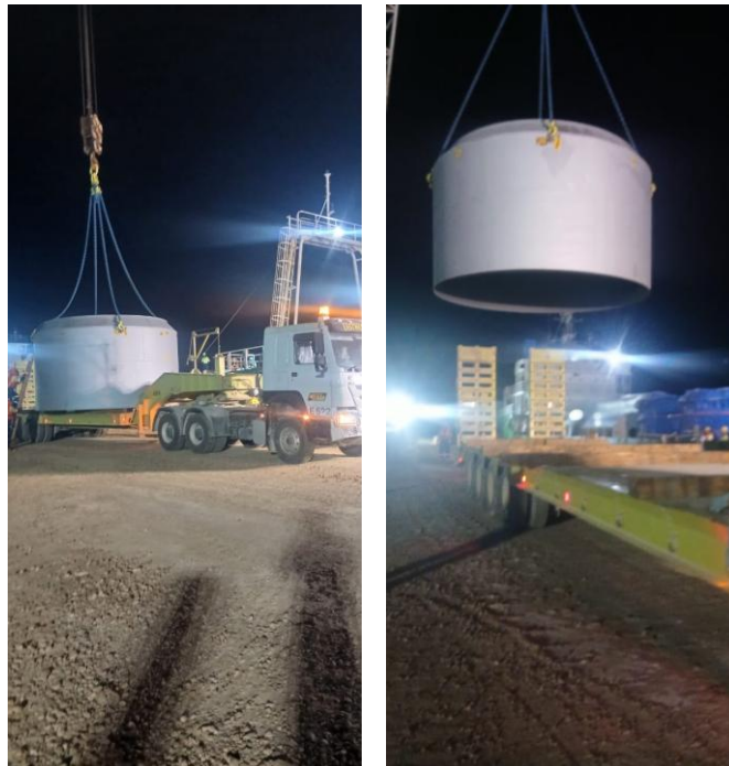
Photo: Landside – first kiln shell sections offloaded from the first shipment being unloaded and transferred to kiln site.
