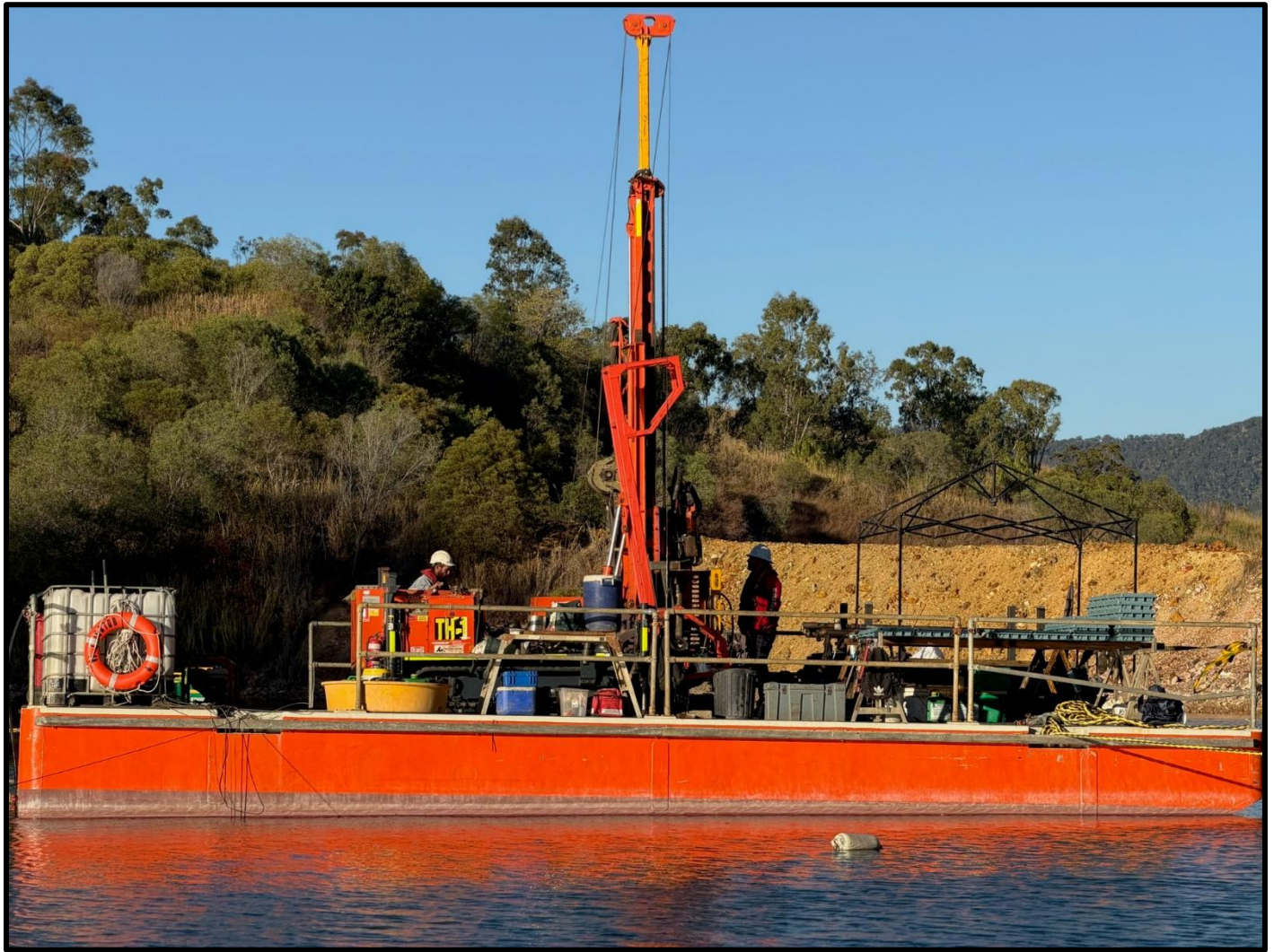
Figure 6 – Rig 19 Barge Drilling.
