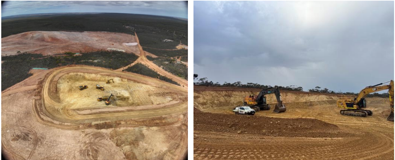
Figure 2: Kundip site infrastructure and preparations for underground mining.
