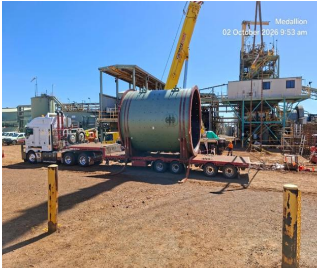
Figure 4: Second ball mill and Carbon in Leach (CIL) circuit foundations at the Cosmic Boy Concentrator.
