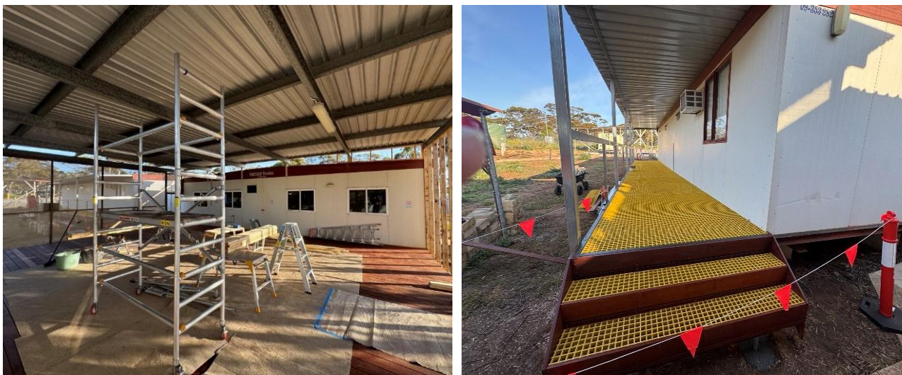
Figure 3: Ravensthorpe accommodation and supporting infrastructure upgrades.
