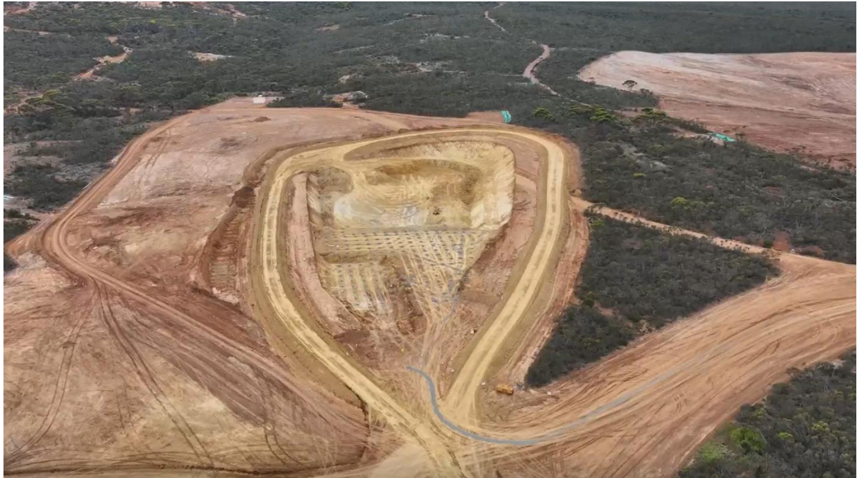
Figure 1: Aerial view of Kundip showing progress across the box cut ROM pad, waste dump and access roads.
