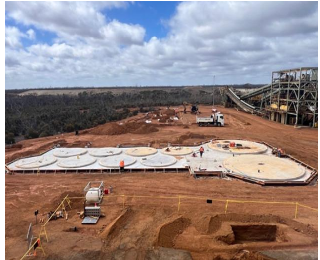
Figure 4: Second ball mill and Carbon in Leach (CIL) circuit foundations at the Cosmic Boy Concentrator.
