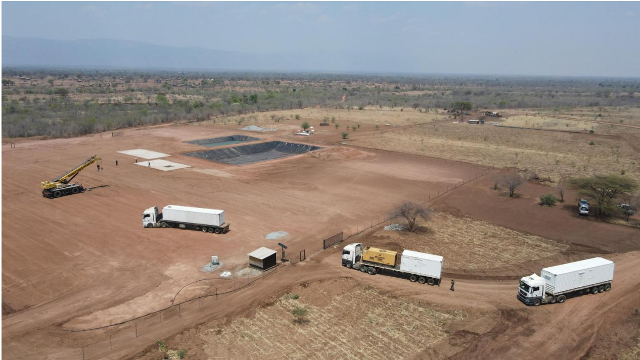
Figure 3 – Arrival of first load of Rig 202 camp
