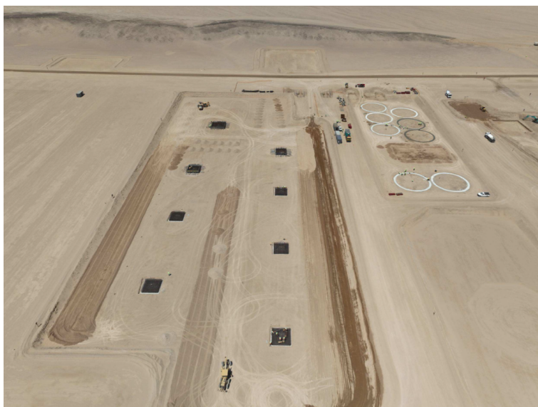
Figure 10: Overall Processing Plant Construction Progress
