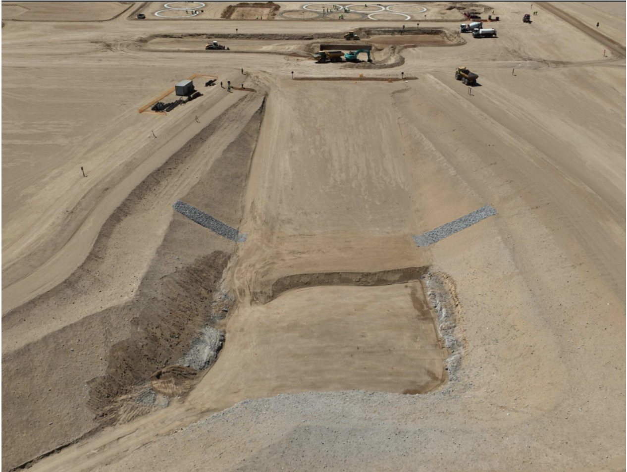
Figure 5: ROM Bin Excavation and Retaining Wall Preparations
