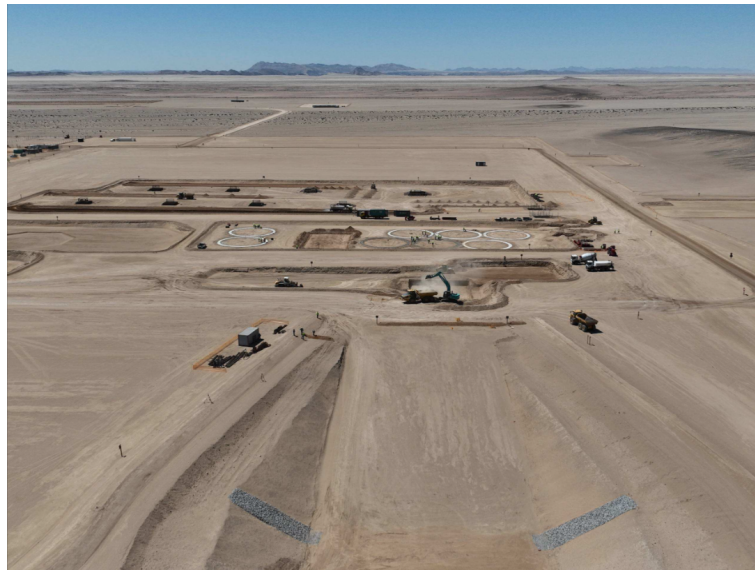
Figure 9: Processing Plant Development – Looking North
