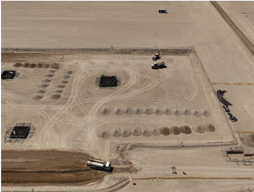
Figure 1: CCD Centre Boss Foundation Preparations
