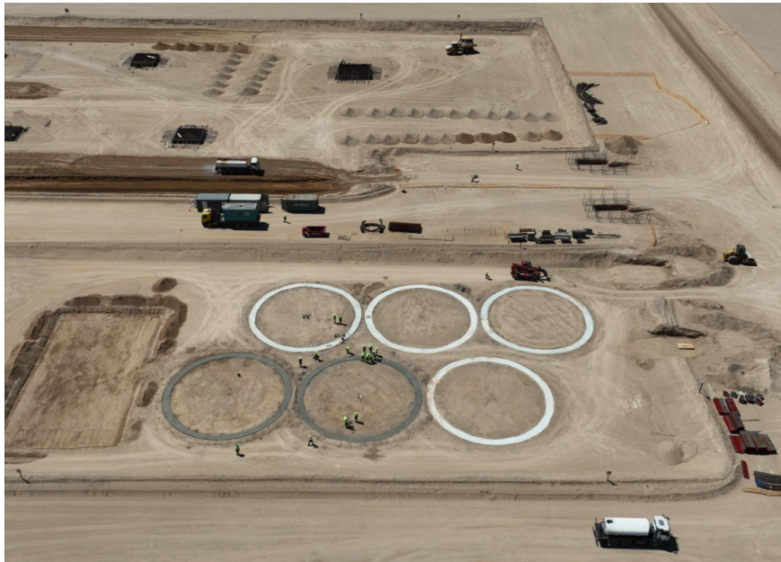
Figure 3: Leach Tank Ring Beam Preparations
