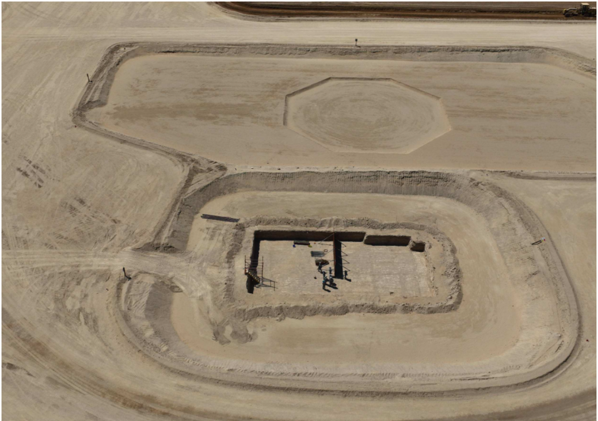
Figure 6: Fine and Coarse Mill Foundation Preparations
