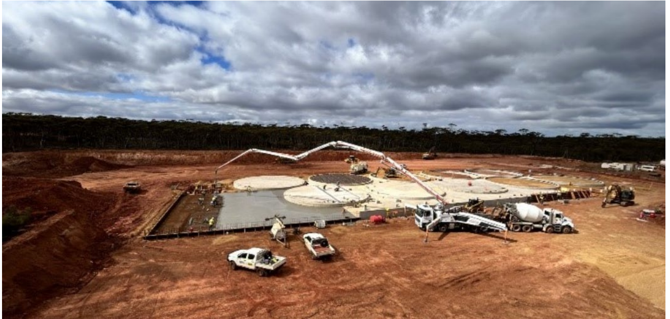
Image 13: Concrete works – CIL tank area – Lake Johnston
