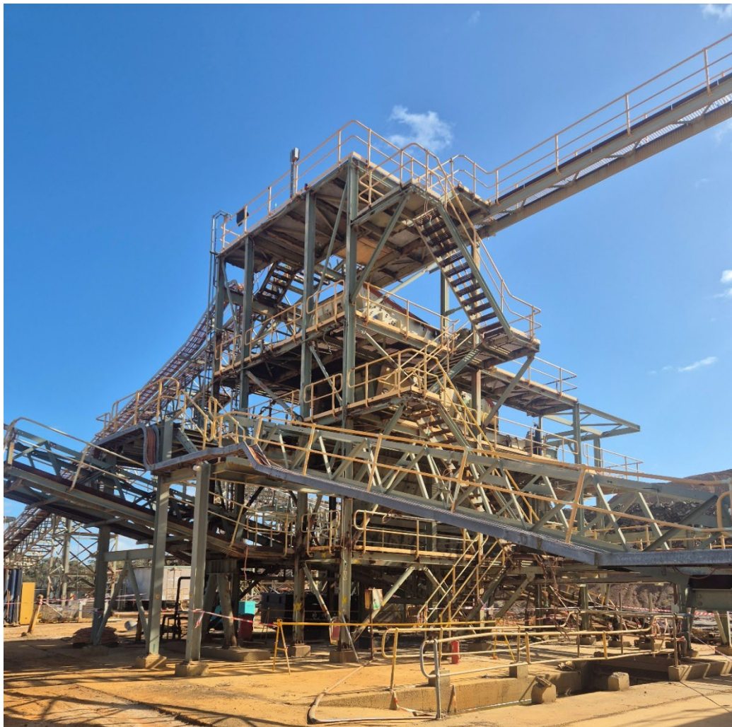
Image 14: Screen tower refurbishment – Lake Johnston
