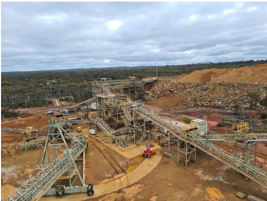
Image 10: Lake Johnston Processing Facility Overview
