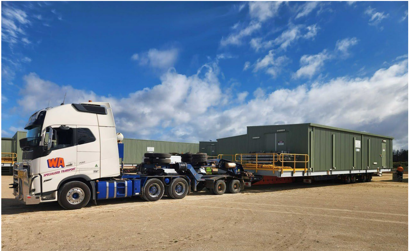
Image 11: Transit of Lake Johnston Motor Control Centre Assembly
