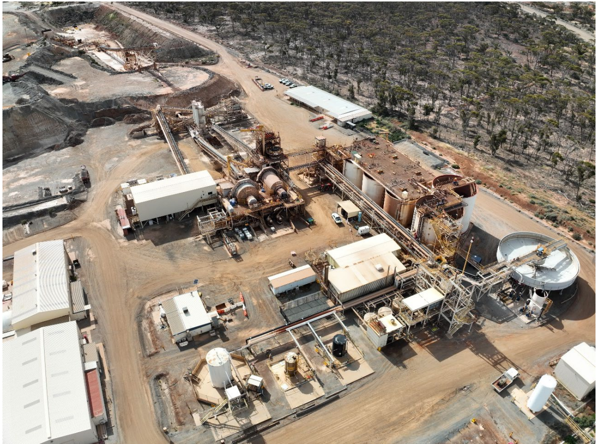
Image 5: Edna May Processing Plant Overview (October 2026)
