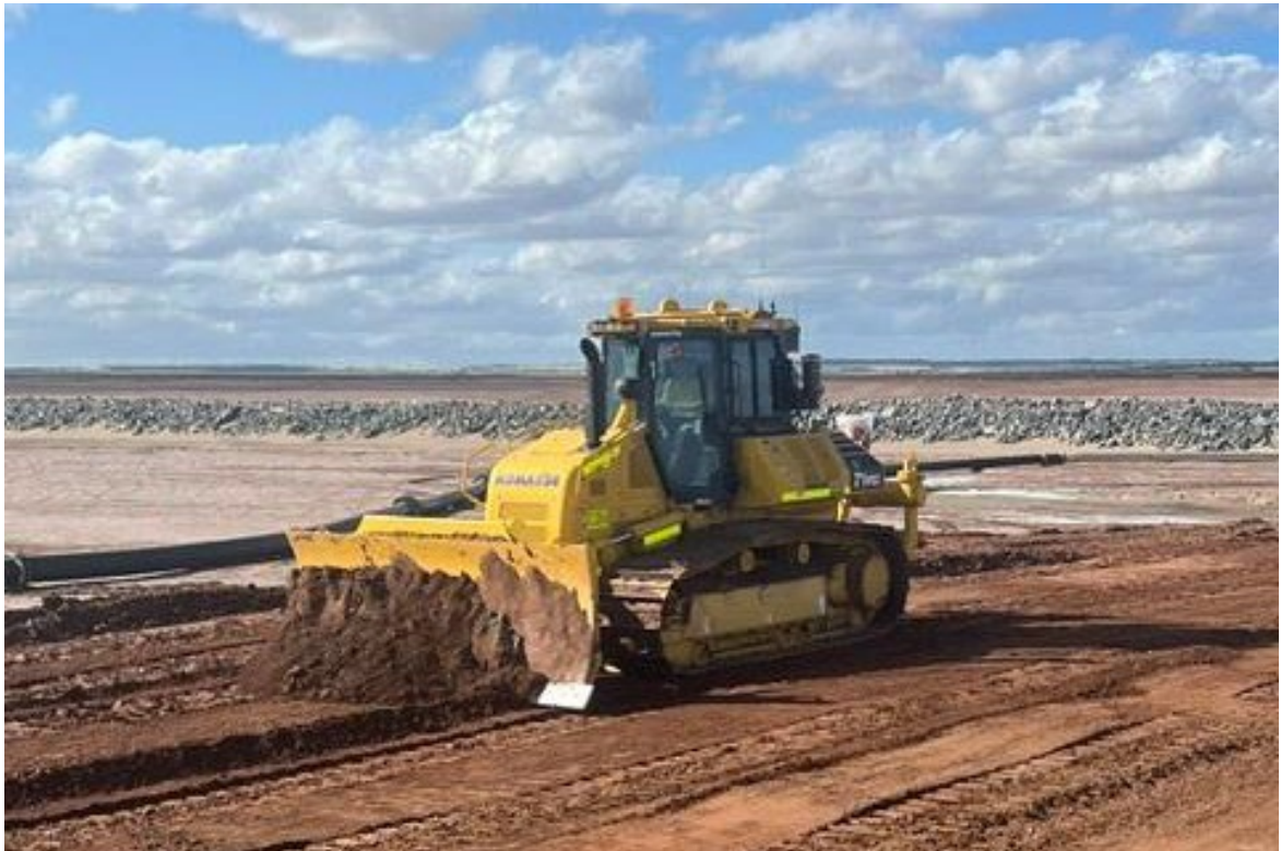
Image 6: Tailings Storage Facility upgrade works – Edna May
