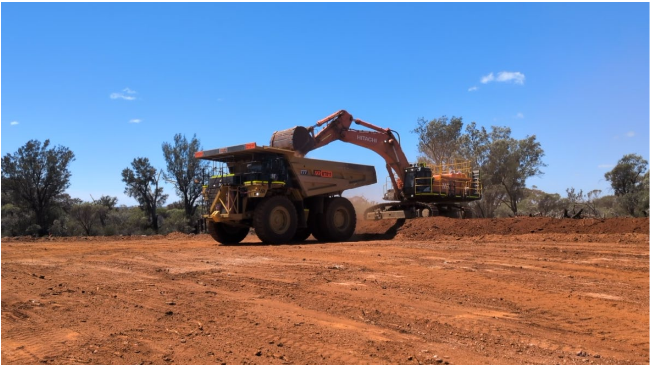
Image 2: Site clearing activities underway – Johnson Range Mine
