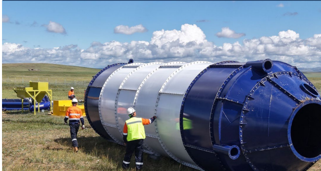
Subcontractor personnel inspecting concrete batching plant equipment delivery
