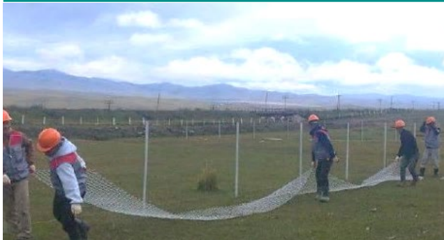
Fence installation at the ERT site around the perimeter of the 30-ha land-use permit
