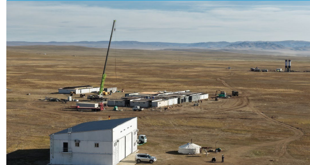
Establishment of site workshop/warehouse and contractor's accommodation
