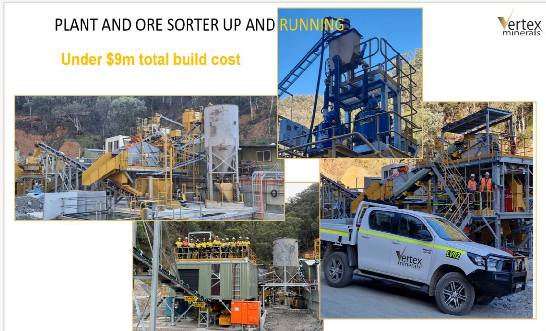
Gekko gravity processing plant, commissioned on site at Reward.
