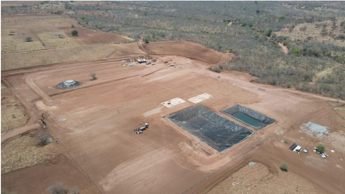
Figure 1 - Musuma-1 wellsite aerial view
