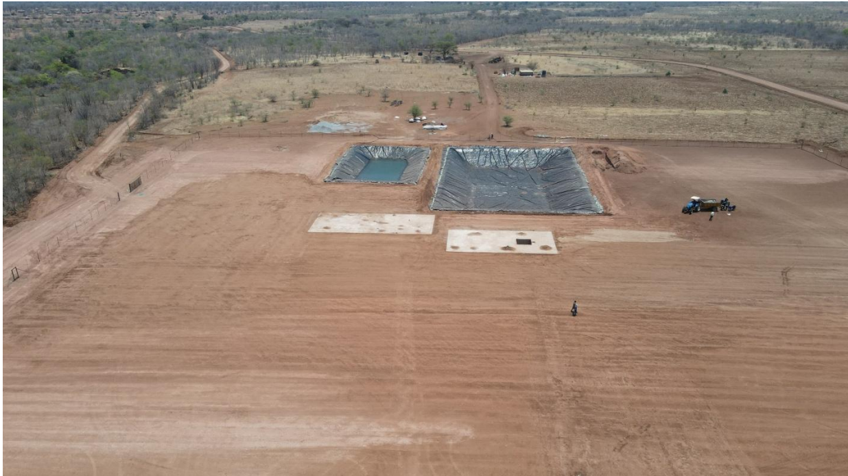
Figure 3 - Musuma-1 rig pad, water supply and waste pit area
