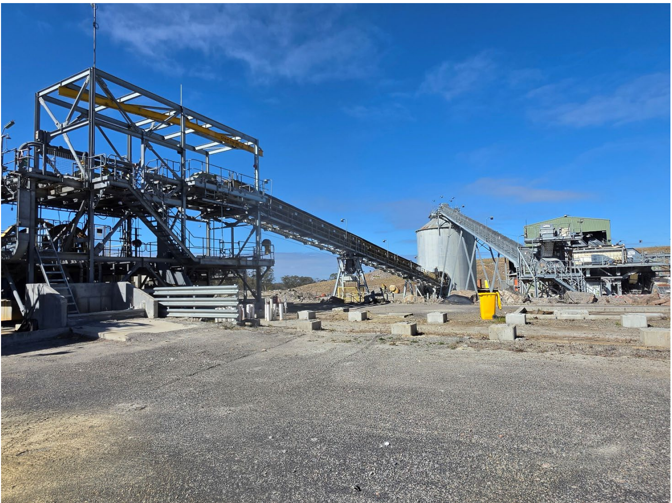
Figure 4. The acquired crushing and processing infrastructure, including mill structure, conveyors and triple-deck screening circuit.
