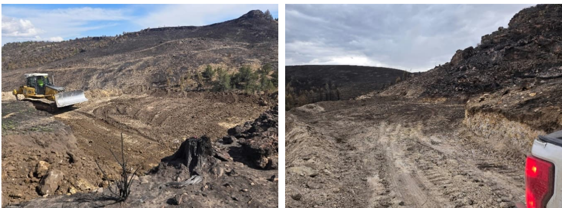
Figures 3-4. Boulder Creek Au-Ag Project – Site Preparation Works for Drilling
