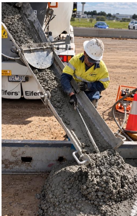
Eifers concrete incorporating G360's MKX calcined clay at Melbourne Airport Business Park, Level Crossing Removal Project and a trial pavement pour at Melbourne Airport.
