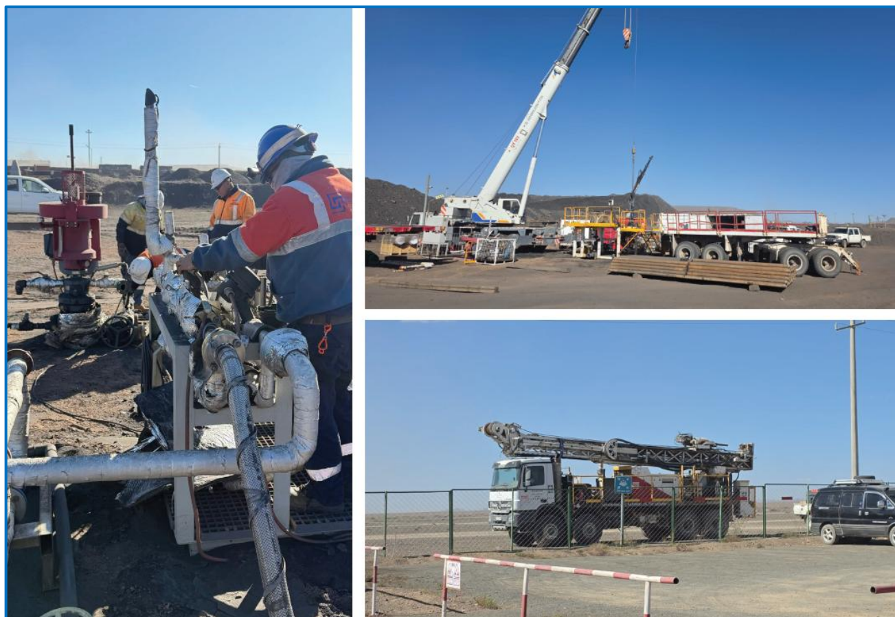
Figure 1: Workover rig arriving at site, 70 tonne crane pulling pump from LF-03 and field staff preparing LF-03 for the workover of the well
