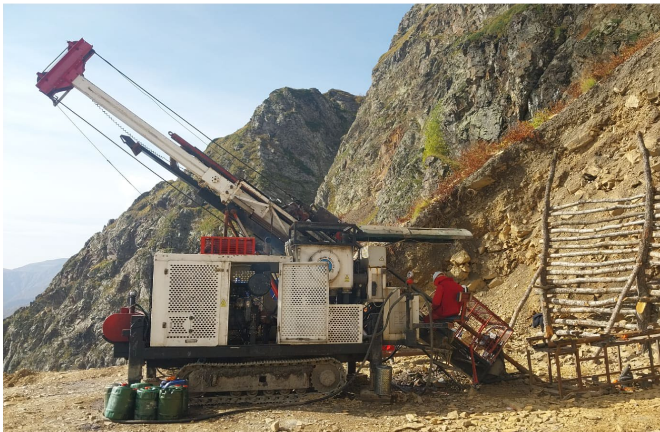
Figure 1 Drill rig on platform 5B at Zopkhito
